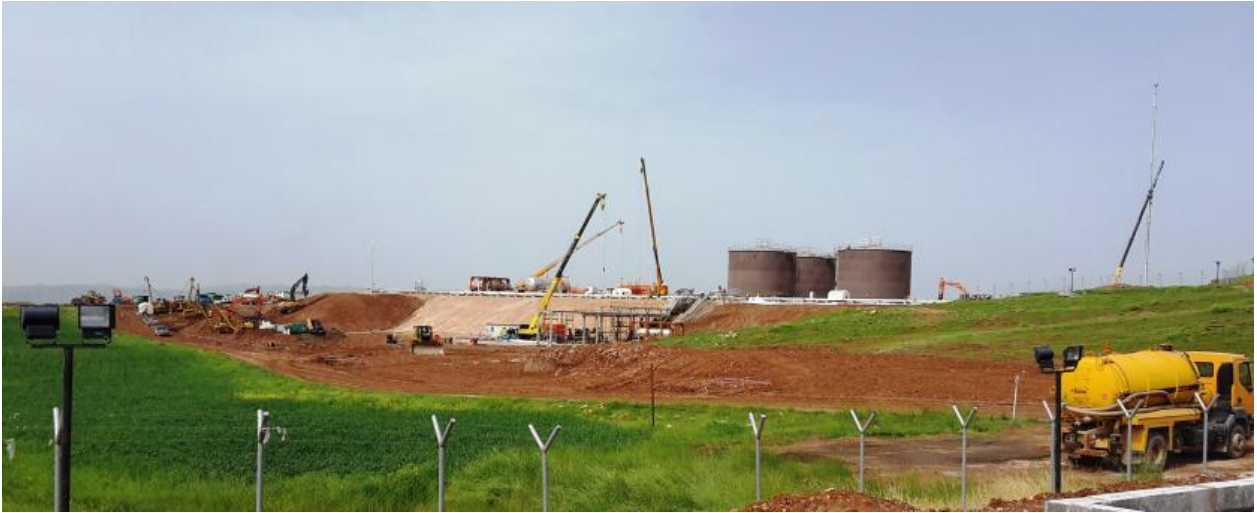
Shewashan EPF under construction – April 2017
